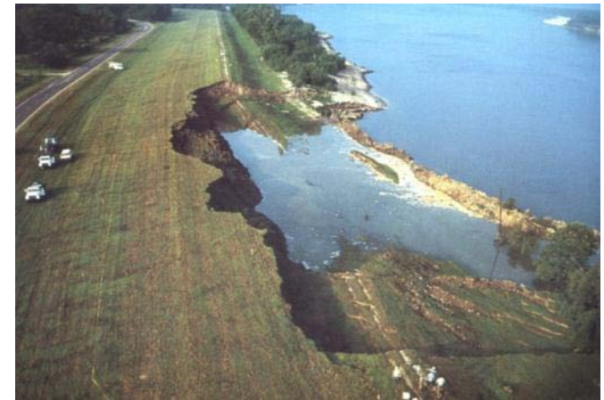
Picture of levee breach
