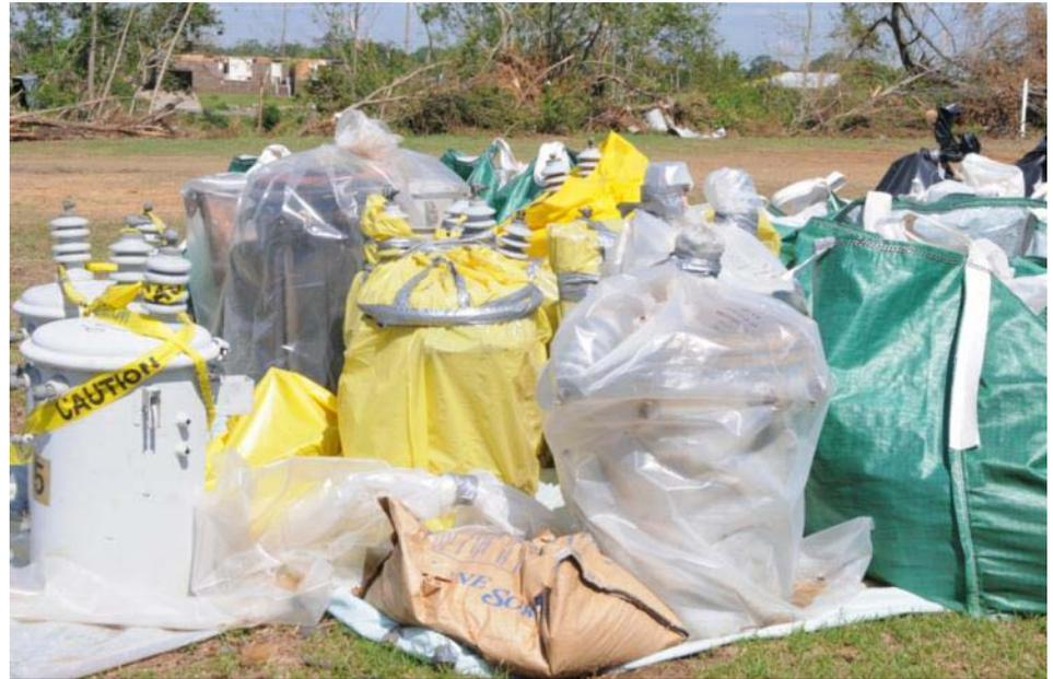
Transformers and other electrical equipment wrapped in bags to prevent oils from leaking
