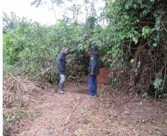
Community members digging a toilet for Ebola Ebola patients
