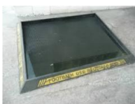
Chlorine foot bath
